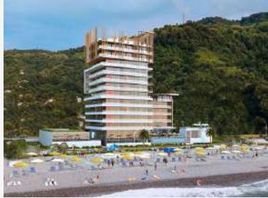
GUMBATI RESIDENCE Gonio, Year of completion 2023
